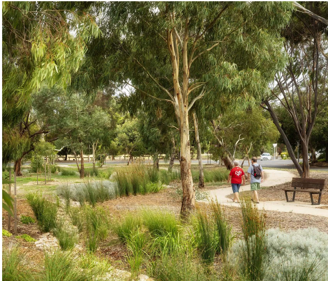
Vegetated detention basin
